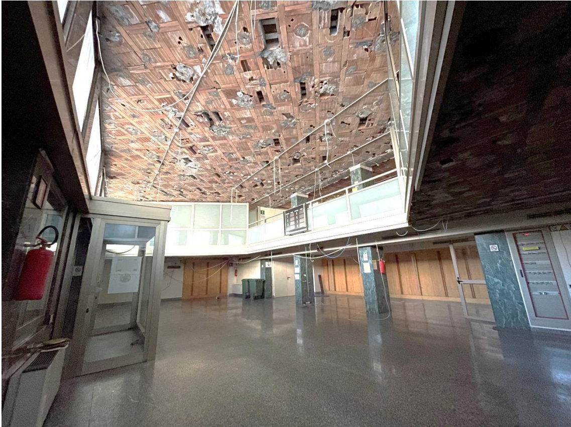
Vista piano terra
