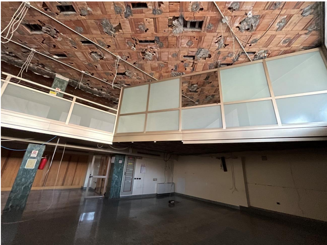
Vista piano terra
