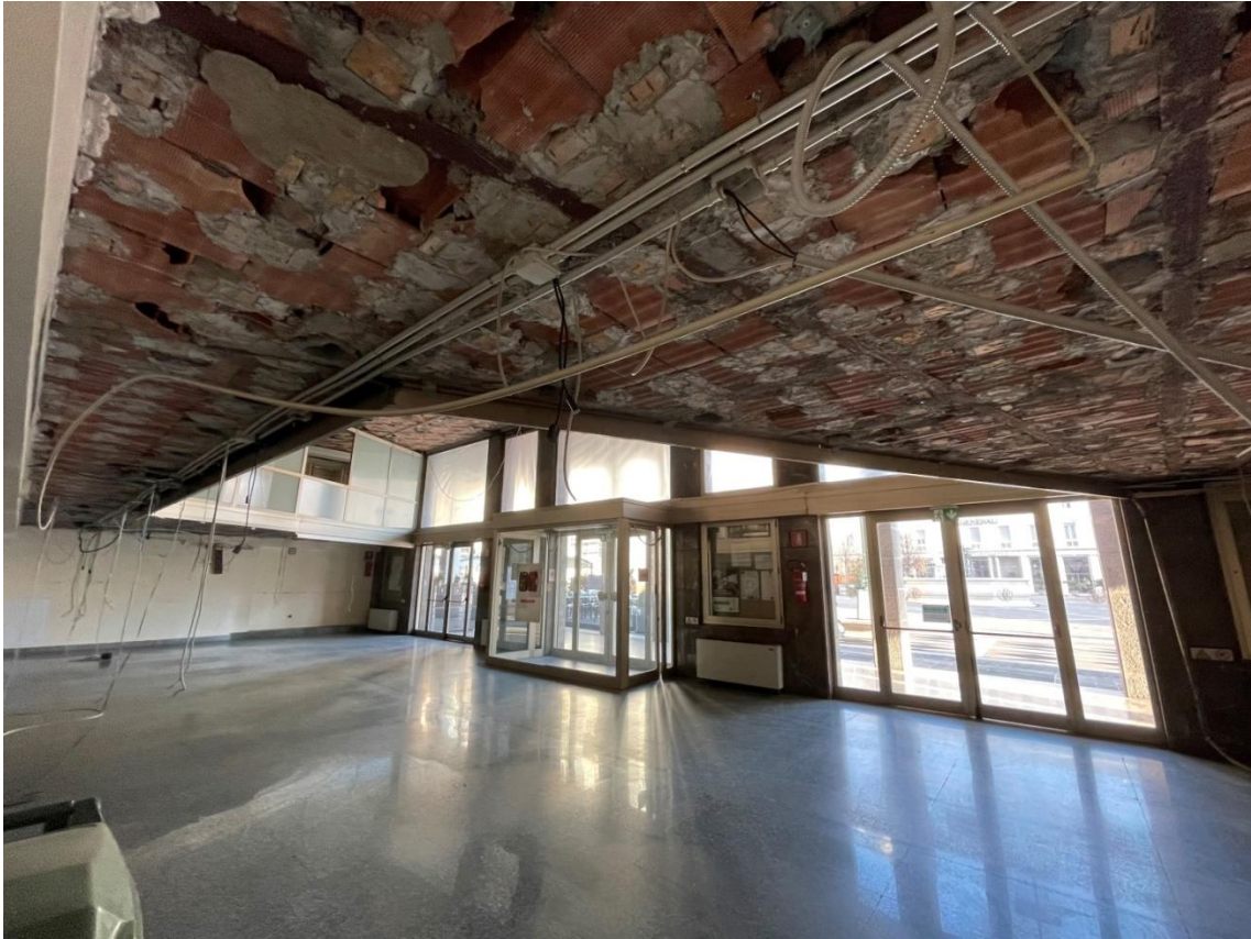
Vista piano terra
