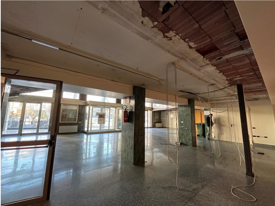
Vista piano terra
